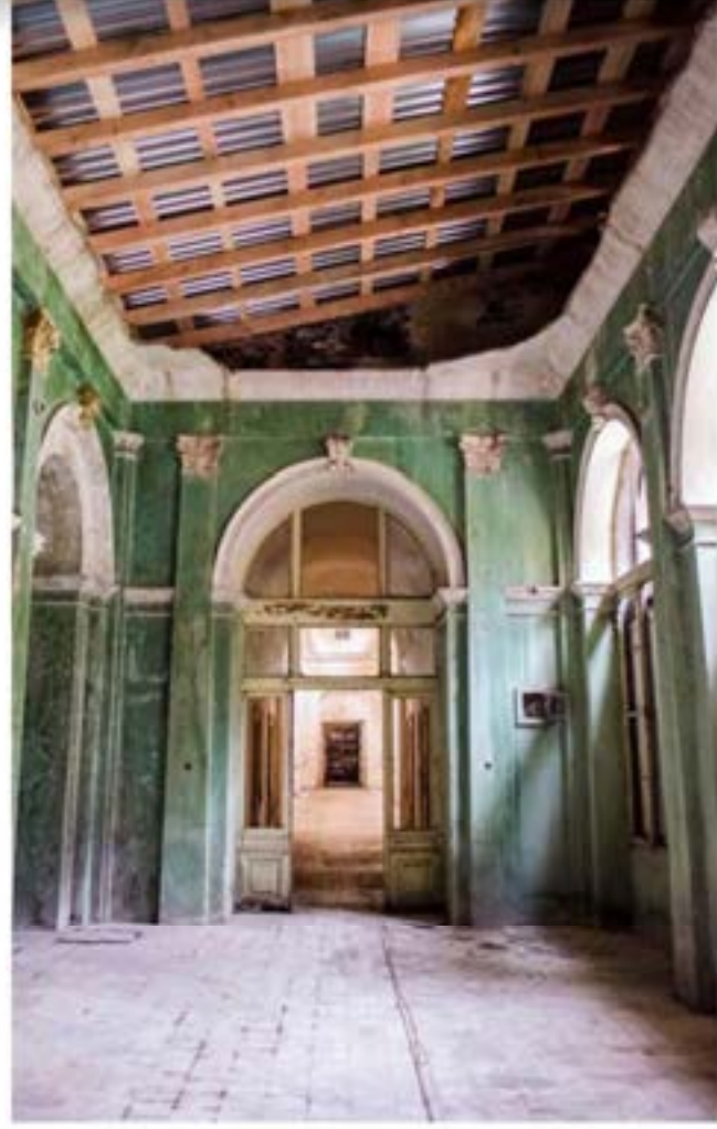
Neptune Baths - construction site for securing the building Photo: Herculane Project, 2019
