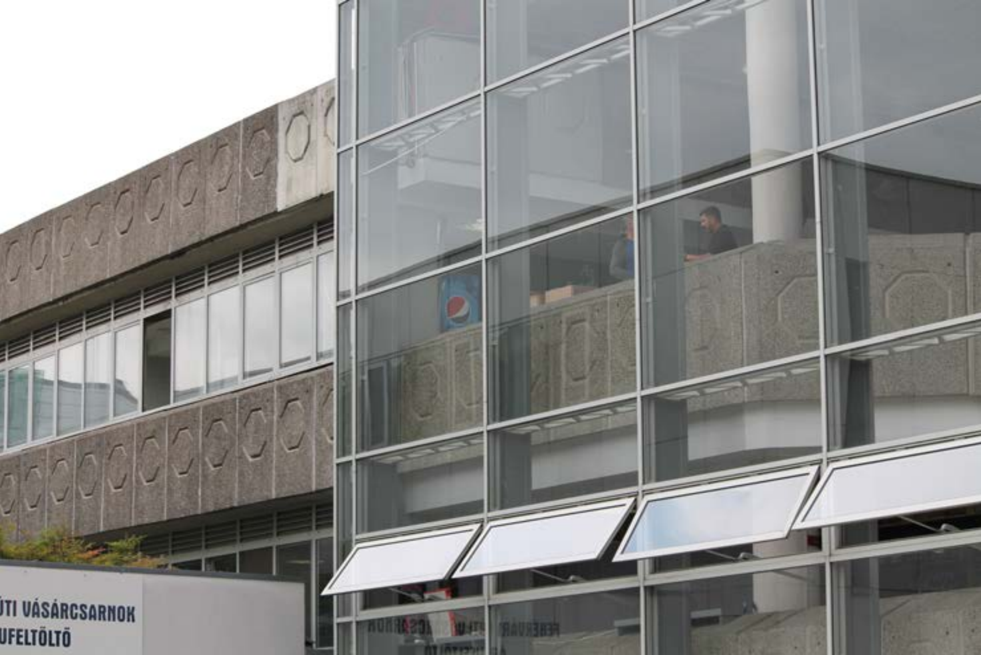
Detail of the market hall today, partially covered and extended
