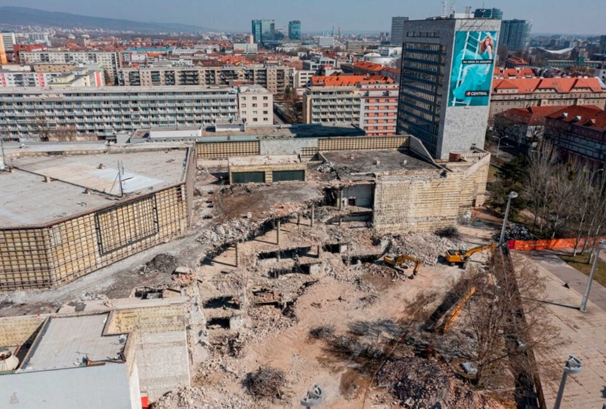
Demolition of Istropolis, currently ongoing
