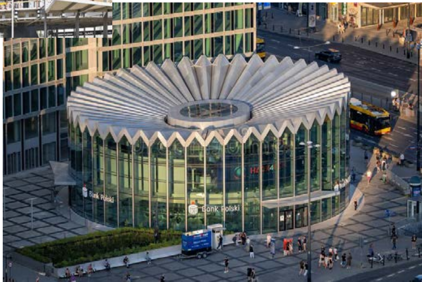
The Rotunda during reconstruction and its current state
