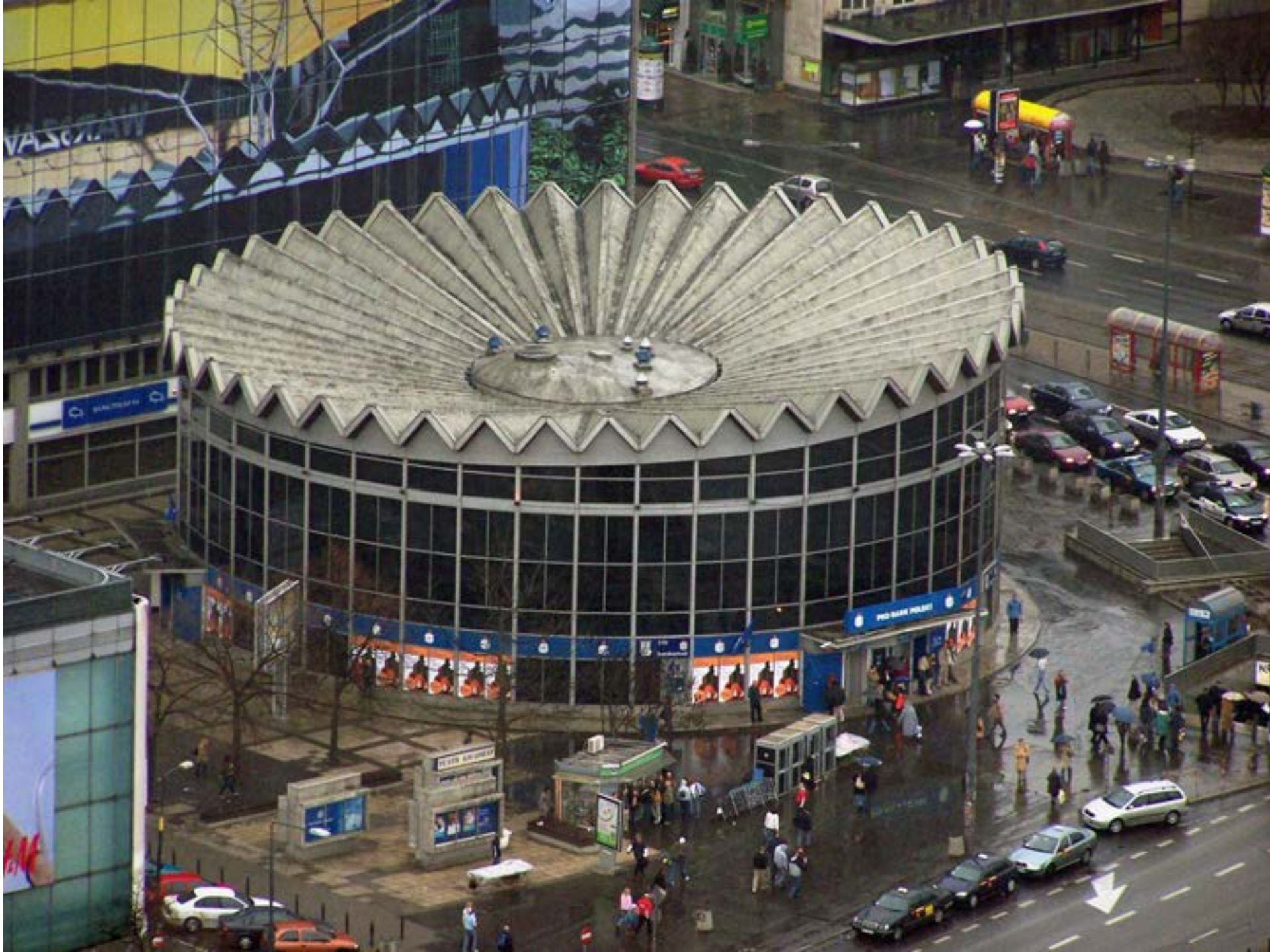
PKO Rotunda, Warsaw. 1960–1969, architect: Jerzy JAKUBOWICZ
