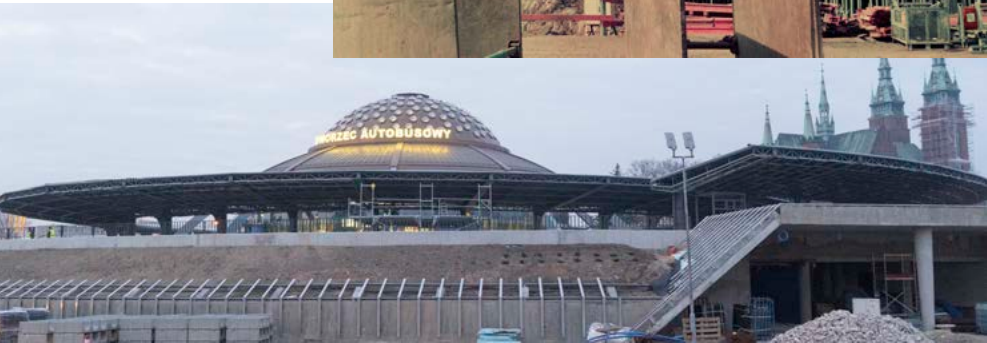
Kielce Bus Station during the renovation work in 2019 and 2020.
