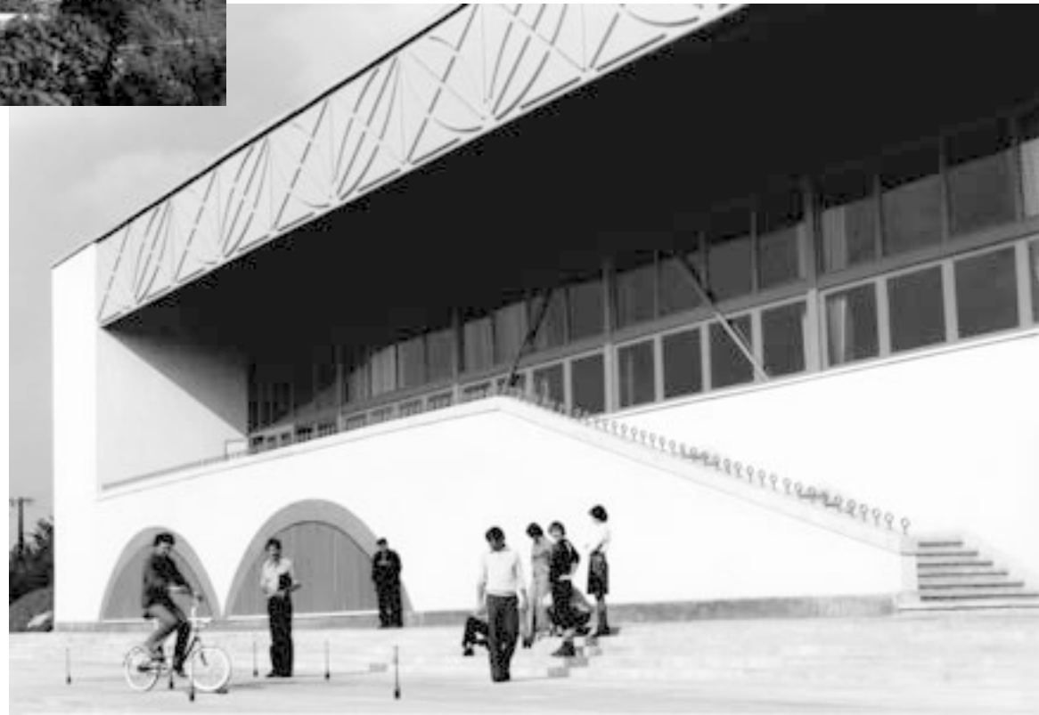
Pioneers' Home in Veszprém, 1982. Architect: ZALAVÁRY Lajos. Demolished in 2008.
