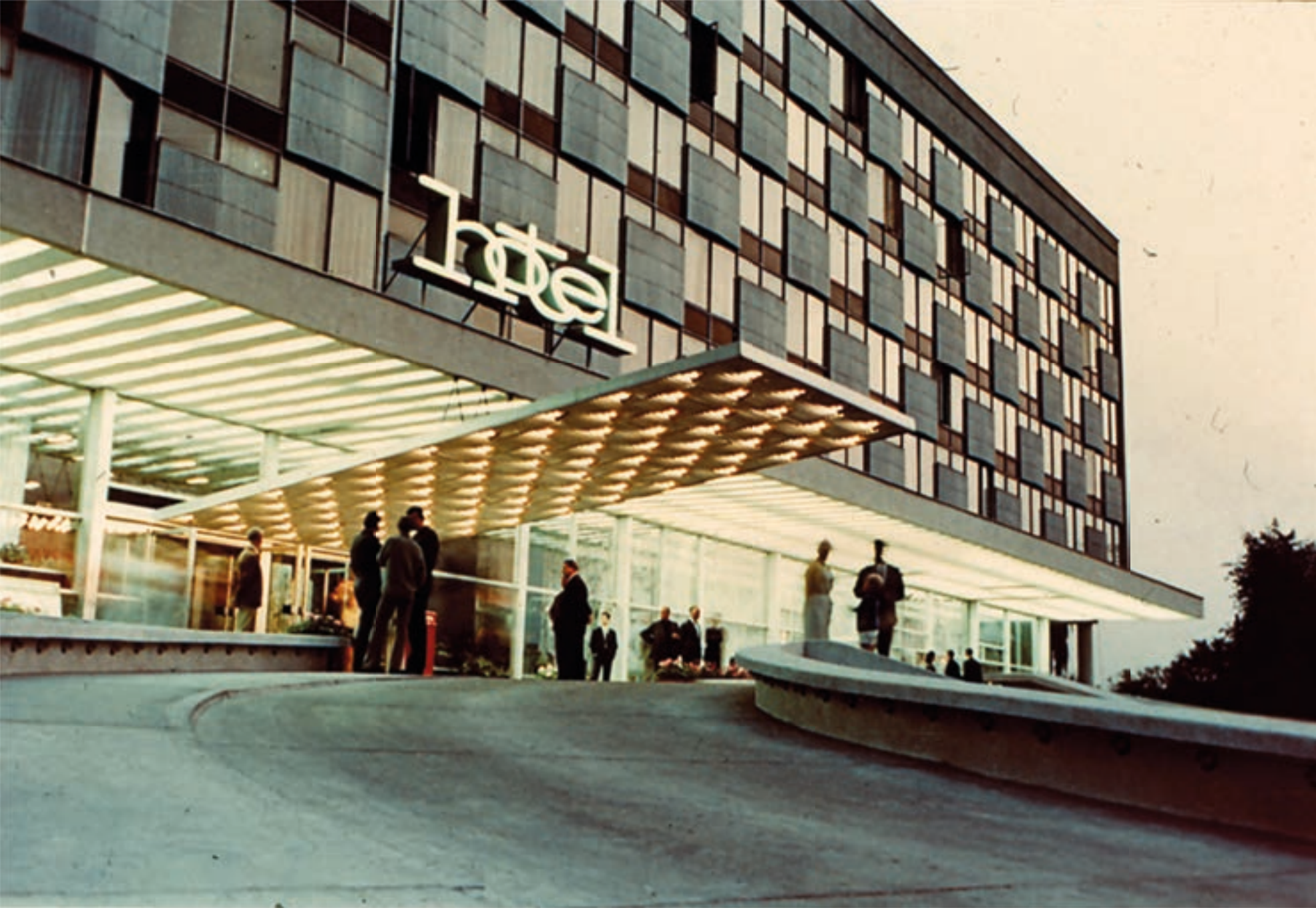
Hotel Cracovia, Krakow. 1960–1965, architect: Witold CĘCKIEWICZ
